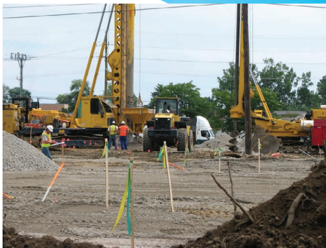
Construction is under way at the Life Time Fitness on Telegraph.
